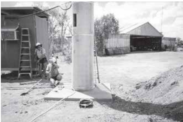
Square excavation around bored hole for collared footing
