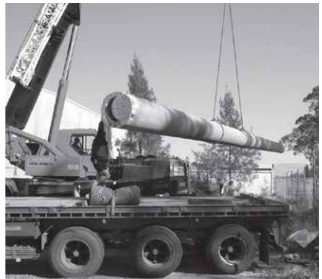
Unloading poles with chain sling
