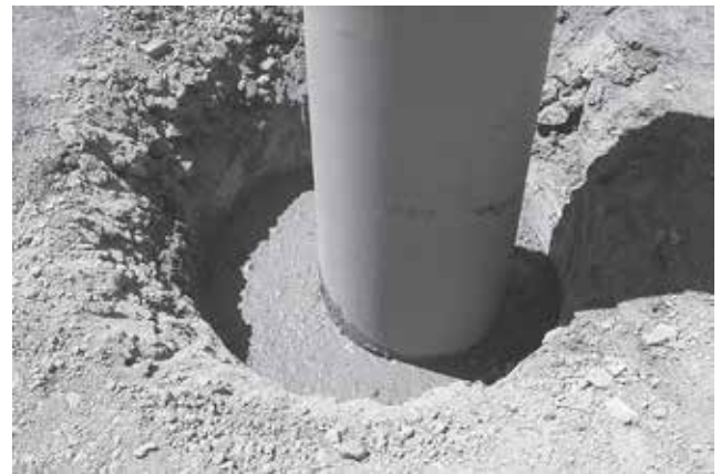
Backfilling with concrete
