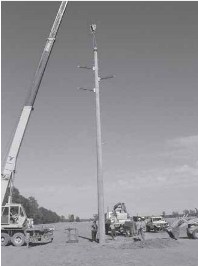
Placing the pole
