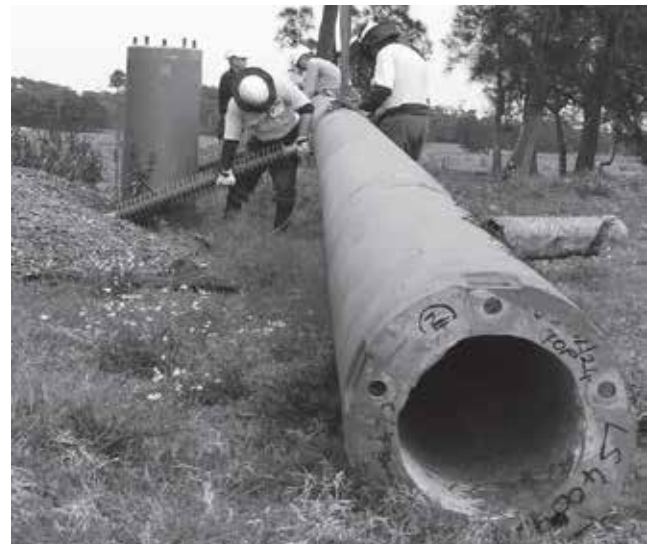
Installing fittings before erection
