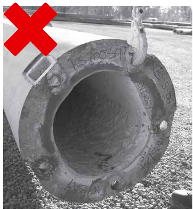
Poles or piles must not be lifted via joint lugs
