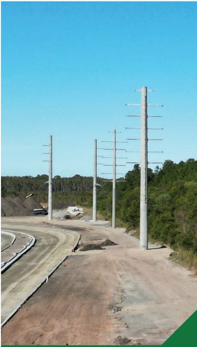
New 132kV Line to Substation Sunshine Coast QLD, Energy Queensland
