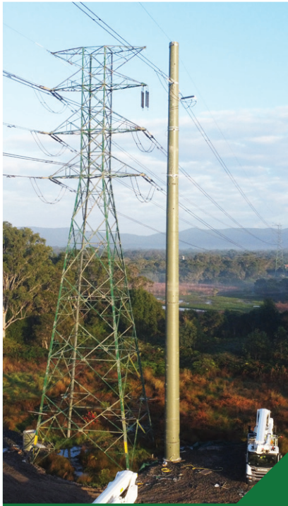
Corroding Lattice Towers Teralba NSW, Ausgrid
